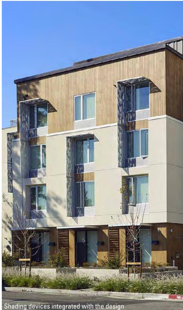
Shading devices integrated with the design
